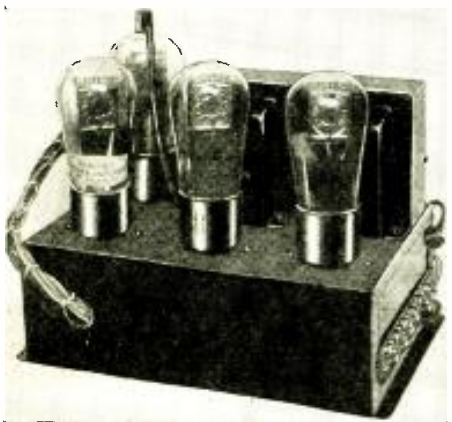
Fig. B Photograph of the amplifier itself. The cable connects to the batteries housed in the case.
